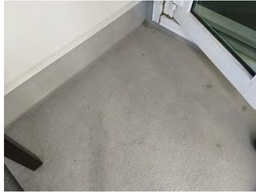
Item 29 - Liquid Applied Urethane Membrane - Balconies
