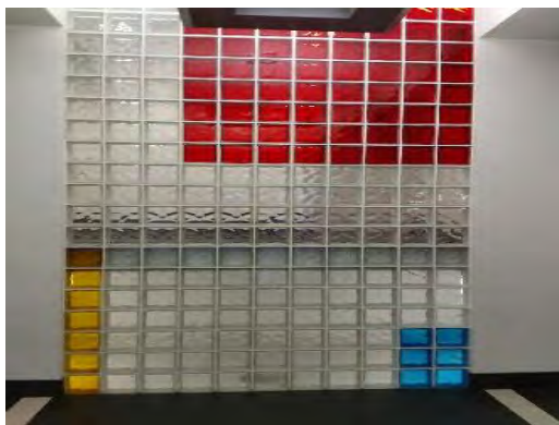
Item 12 - Glass Block Masonry
