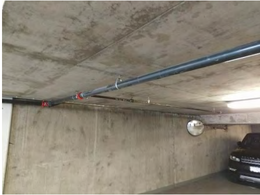
Item 1/2 - Below grade foundation walls
