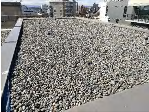
Item 28 - Low Sloped Main Roof Membrane
