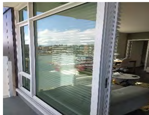
Item 17 - Window Wall Assembly
