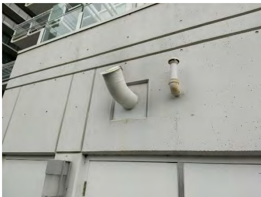
Item 8/15 - Painted Concrete
