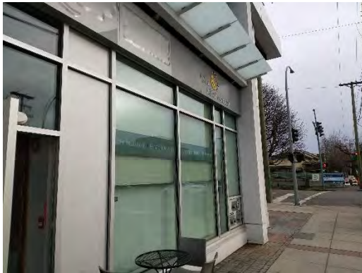
Item 19 - Storefront Curtain Wall
