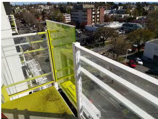
Item 6 - Aluminum Railings w/ Glass Panel
