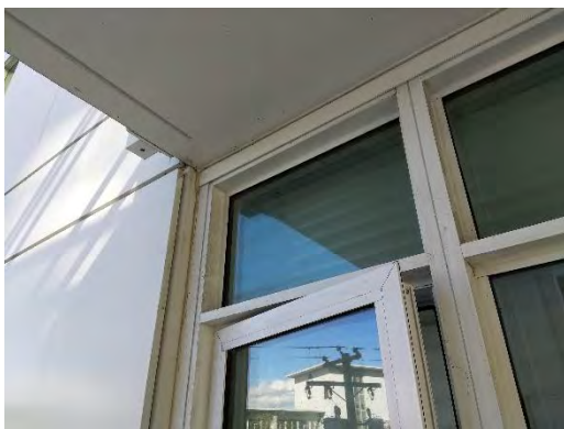
Item 16 - Joint Sealant
