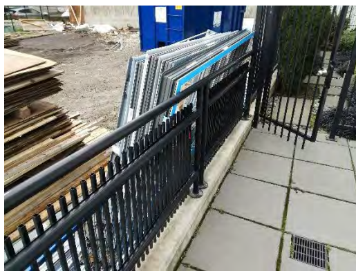
Item 65 - Guardrails and Barriers
