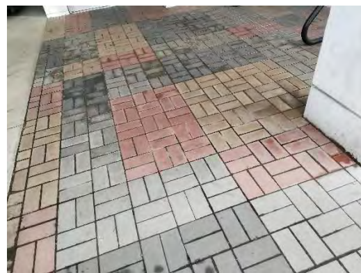
Item 66 - Pedestrian Paving
